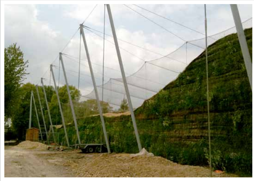
Illustration of an option for mast and tie back design.
