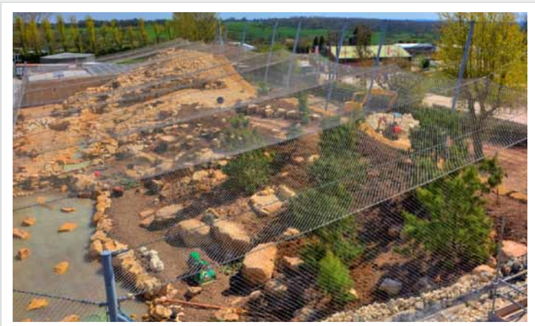
Enclosure side view of the net structure and cable supporting structure illustrated in the previous photograph.
