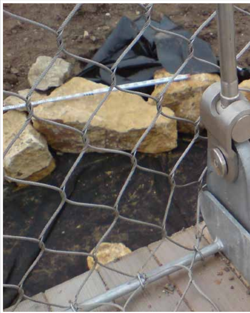
Above: 75 x 75 x 3.5 mm woven/spliced stainless steel net
